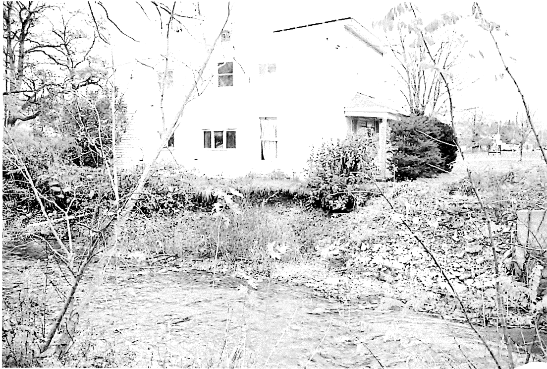
Picture #3 - Eroded banks along White Creek; facing north
