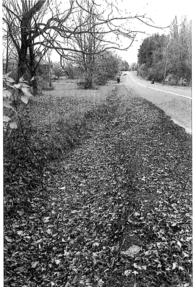
Picture #7 - Undersized, over vegetated ditching; facing north
