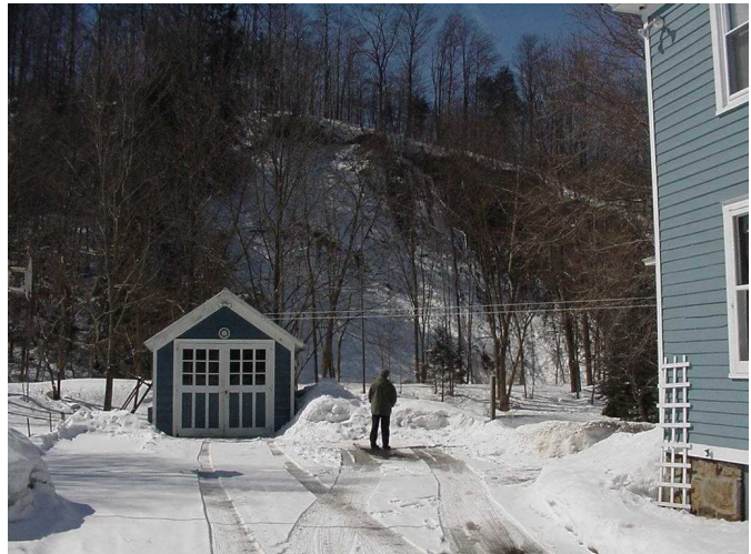
Figure 3: Severe bank slump behind the Bielanski residence.
