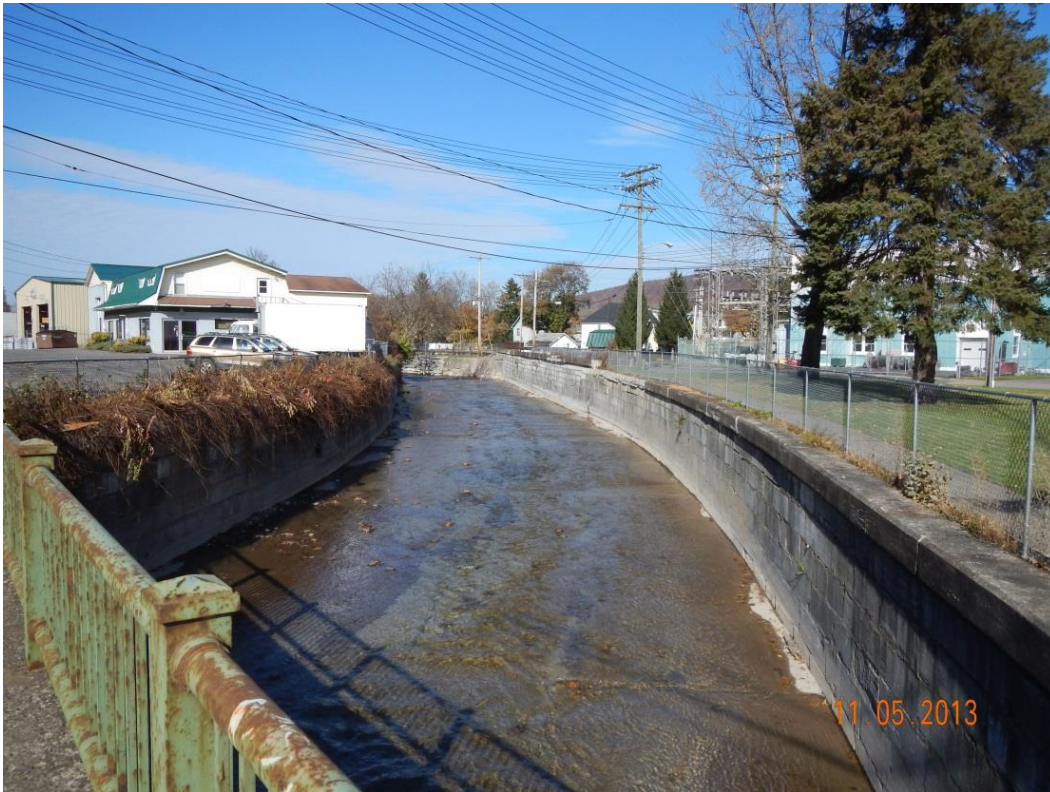
Photo Source: Milone & MacBroom, Inc. (2013)
