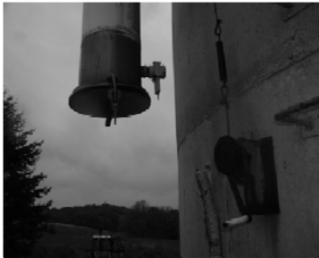
Breather tube connection to fill pipe
