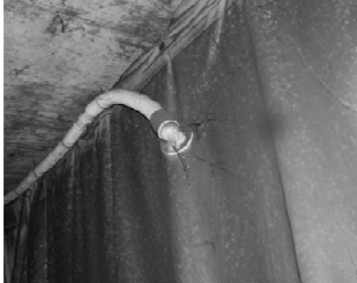
Breather tube connected to breather bag
