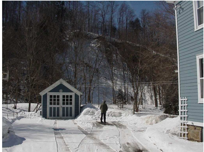
Figure 3: Severe bank slump behind the Bielanski residence.
