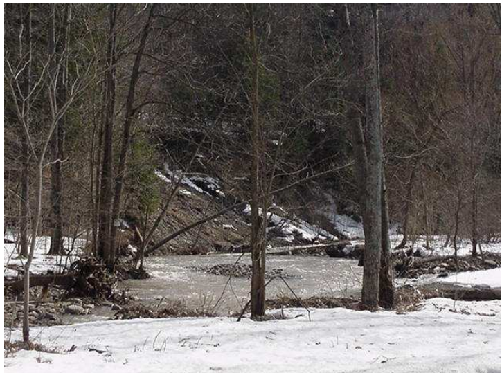
Figure 20: Bank slump near Fox residence.
