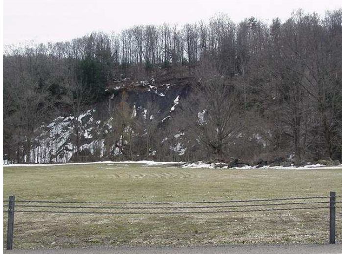
Figure 16: A severe streambank slump on the eastern bank of Moyer Creek.
