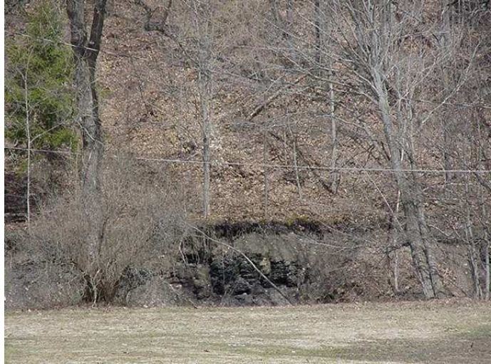
Figure 7: (Above) Northern most bank cut near Casey Road.
