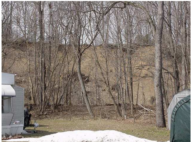
Figure 15: Erosion near Edgebrook Estates in Frankfort.
