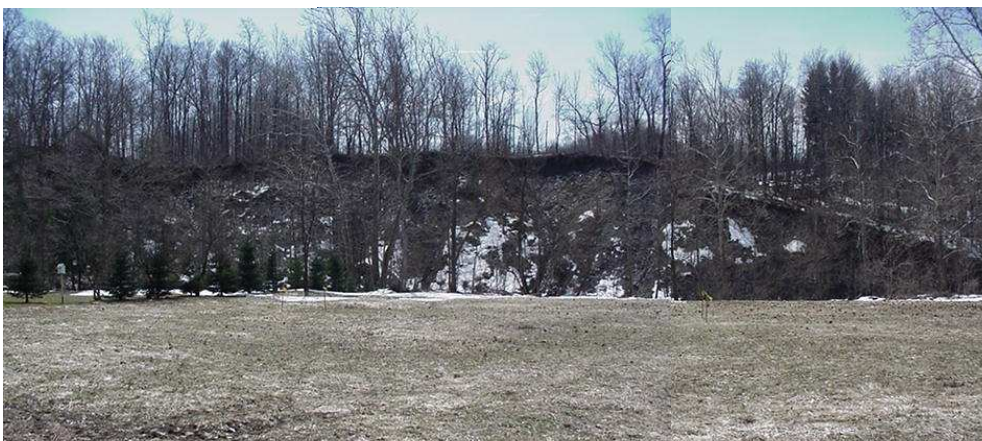
Figure 11: Severe bank erosion near Rock Hill Road
