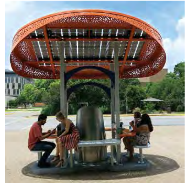
Campus Solar Charging Station https://www.soldesignlab.com/
