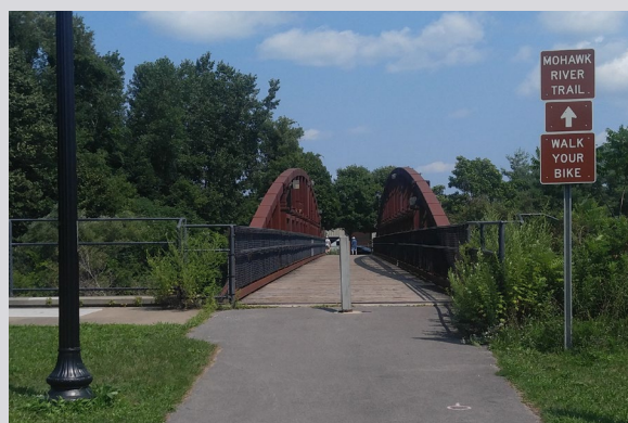
Bridges allow bicyclists and pedestrians to cross the Canal.
