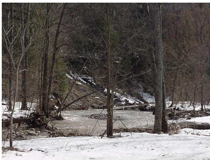
Figure 20: Bank slump near Fox residence.
