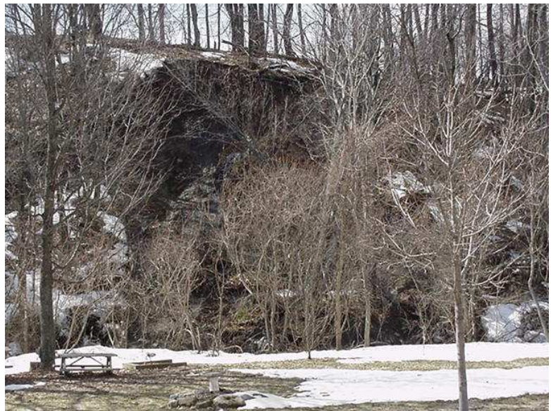
Figure 12: Stream bank erosion near McCready Road
