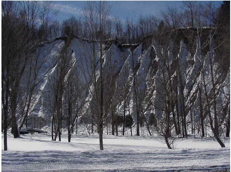
Figure 9: Most severe bank slump on Fulmer Creek.
