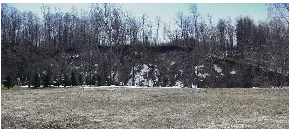
Figure 11: Severe bank erosion near Rock Hill Road
