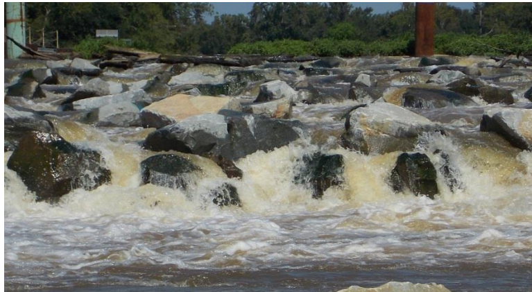
FIGURE 8 Example Rock Ramp
