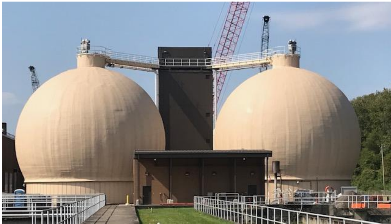
Figure 3. New egg-shaped digesters and septage receiving station at the Oneida County Water Pollution Control Plant. Source: Oneida County.
