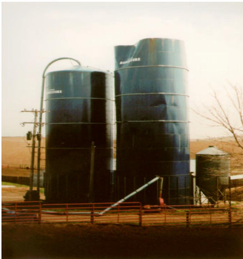
*Deformity of silo shell due to explosion*
